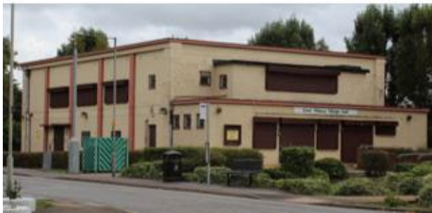
Figure 24 & 25: Bata Cinema © Bata & East Tilbury Village Hall
