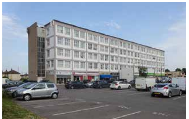
Figure 30: Car Park at Stamford House
